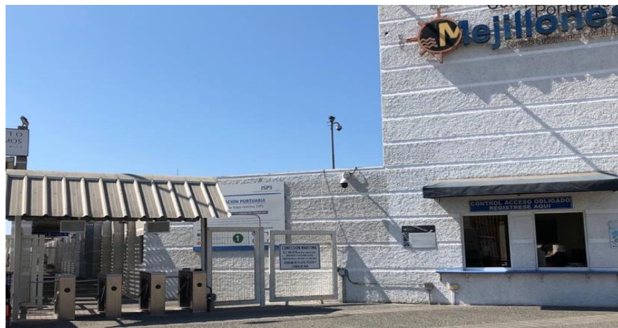
Main Access Puerto Angamos (Turnstiles and Service Window)
